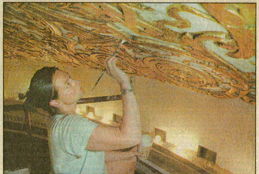
On a platform 60 feet high, Kim Stephenson touches up the paint around some freshly gilded flourishes decorating Proctor's Theatre in Schenectady.
